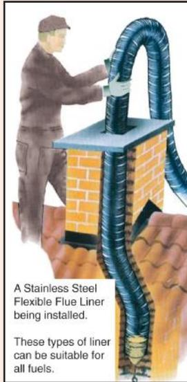
A Stainless Steel Flexible Flue Liner being installed.
