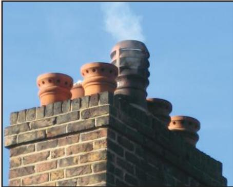
**WARNING** - the chimney termination covers below are only designed for **disused** flues. They are not approved for working gas, oil or solid fuel chimneys.
